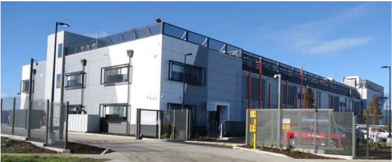
Metronode Data Centres
