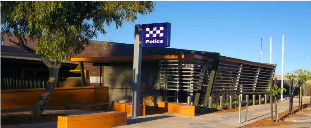
Fitzroy Crossing Police Station
